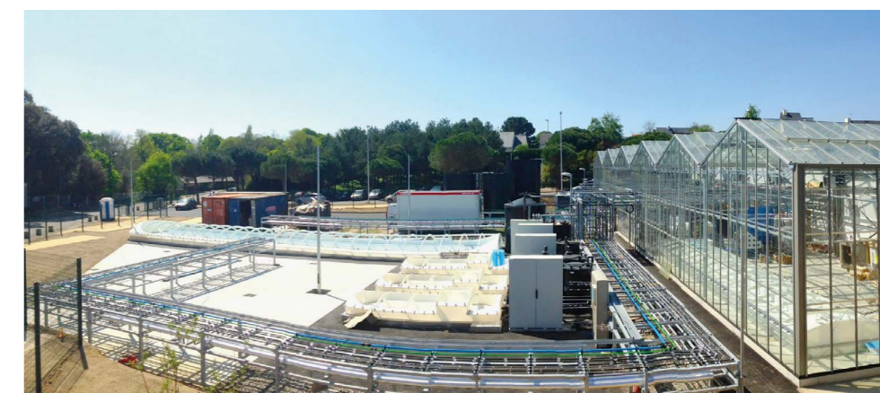
The AlgoSolis R&D facility © GEPEA -Algosolis
